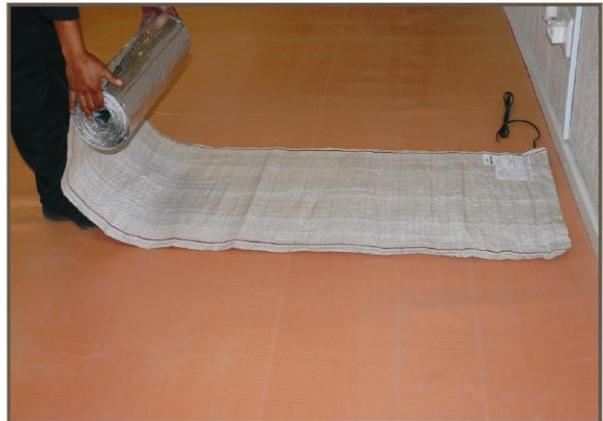
**Carpet heater is secured down with tape.**
