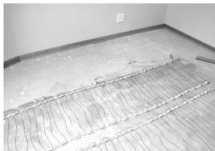
3. Pull the wax paper backing off the tape a little at a time and, keeping it straight, stick it to the floor.
