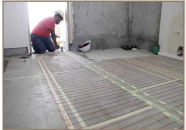
Adhesive mesh is laid on top of the heating element.
